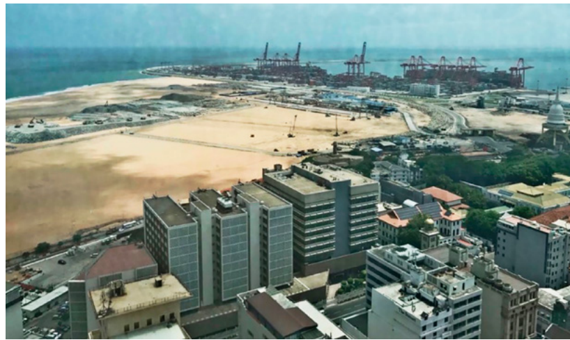
Colombo Port City under construction (Image: Liu Qin)
